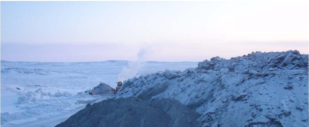
Photo 2 (top center): ~E view of FCM stockpile at the FCP Pad. Note that the frozen material is trying to be seperrated out and the better quality material stockpiled (i.e. small stockpile starting at the forefront of this picture).
