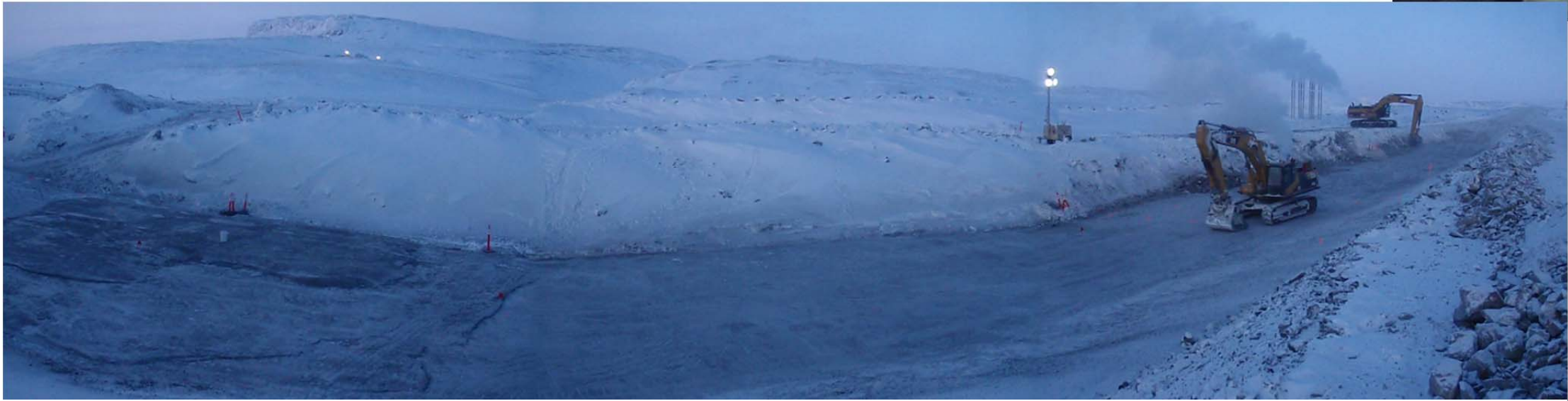
Photo 9: ~ N view of excavators working on cleaning eastern portion of key trench (stitched Panoramic view)
