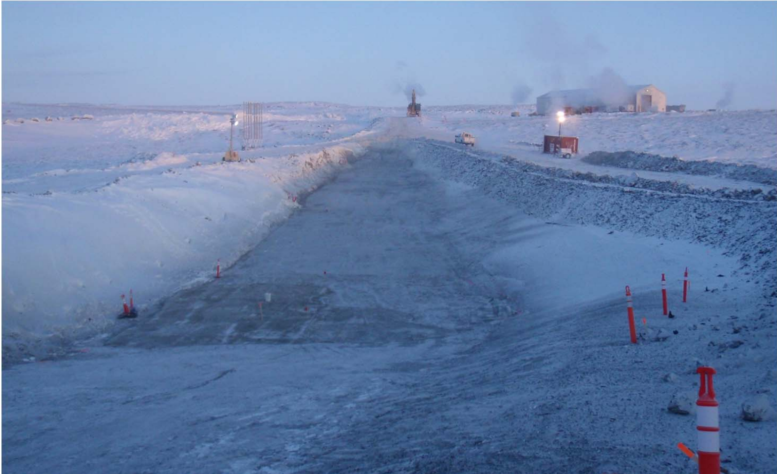
Photo 8: ~ NEE view down key trench. Note recent January 19 th placement is the darker coloured material in the central area.
