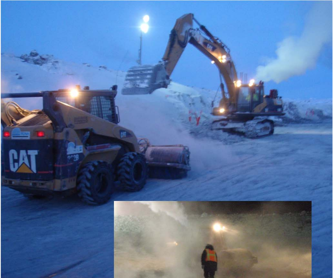
Photo 10 (top right): Bobcat and 330 excavator working cleaning snow and 5/8" material from downstream of key trench.
